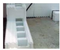
Figure 3: The 'Super R' block in position.
