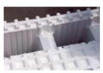
Figure 4: Reinforcement can be inserted on a moulding in the blocks.
